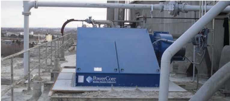
CPV - Multiple Cement Silos 4,800 cfm (8,154 m 3 /h)
