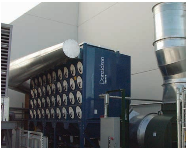
DWS on Custom Hand Grinding 38,500 cfm (65,398 m 3 /h)
