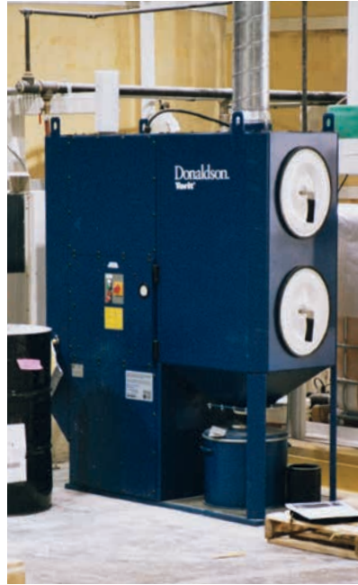
DFO on Paint & Pigment 1,200 cfm (2,038 m 3 /h)
