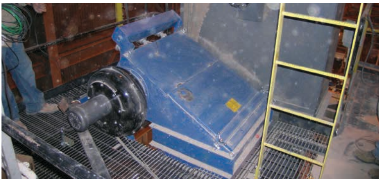
CPV - Bucket Elevator 1,200 cfm (2,038 m 3 /h)
