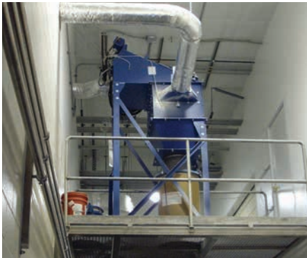
CPC on Milk Powder 1,200 cfm (2,038 m 3 /h)
